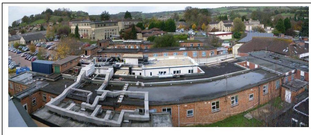
Fig E: View of existing RUH North blocks
