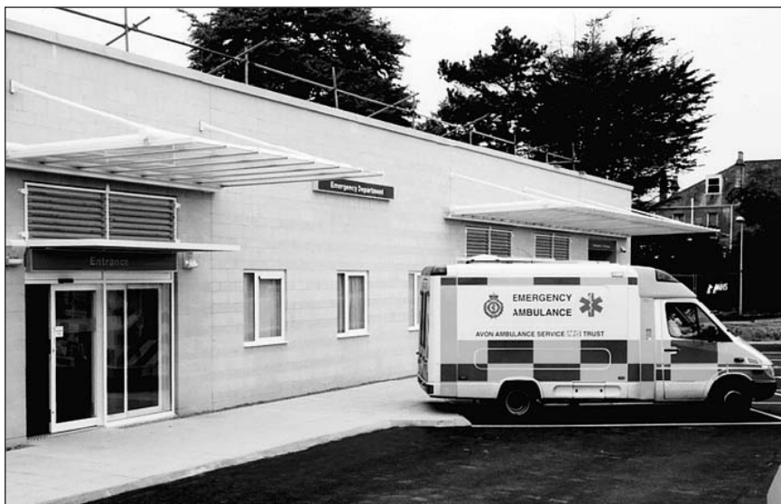
At the end of the year work was nearing completion on a new purpose built emergency department
