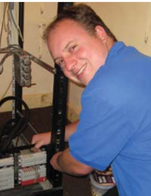
Station engineer Tom Scott working on the replacement broadcast communications tower
